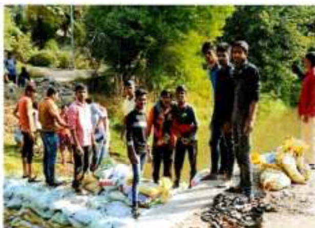
Construction of Vanrai Dam
