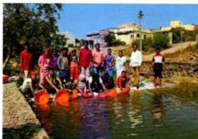
Construction of Vanrai Dam
