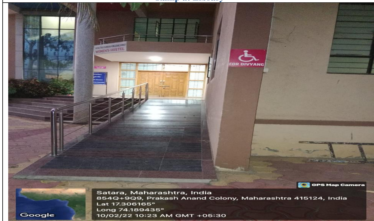
Ramp at Women's Hostel
